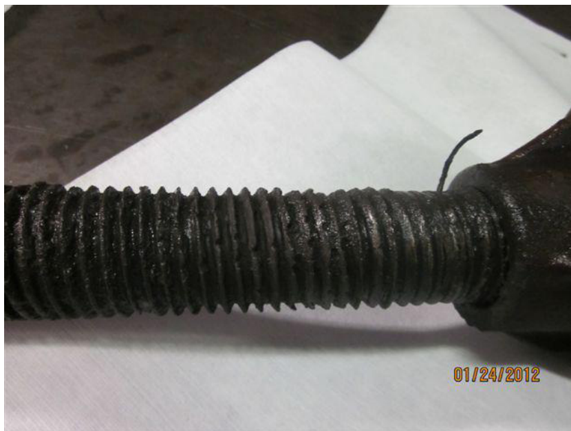
FIGURE 6.13. CORRODED LANDING LEG SCREW (PHOTO FROM [126])
