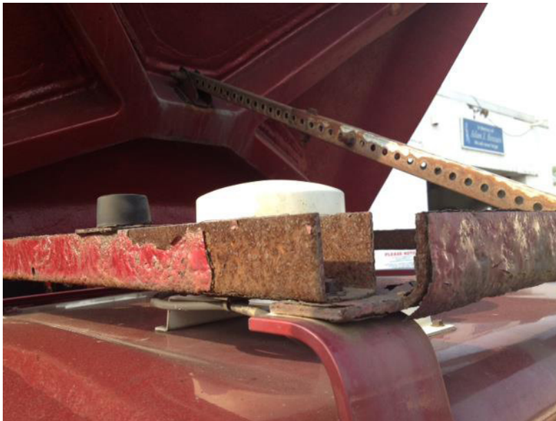
FIGURE 6.12. CORRODED AIR SHIELD SUPPORT FRAME (PHOTO FROM [126])
