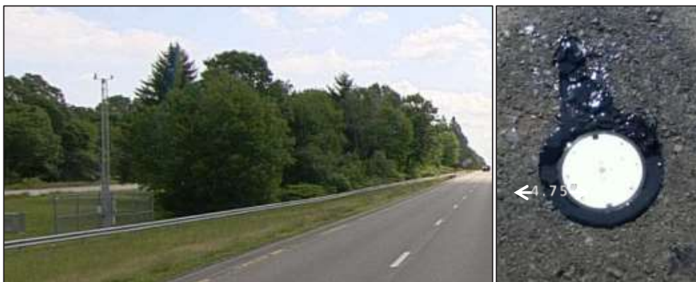
Figure 2: RWIS: Station, Route 2, Lebanon, CT (Left)
