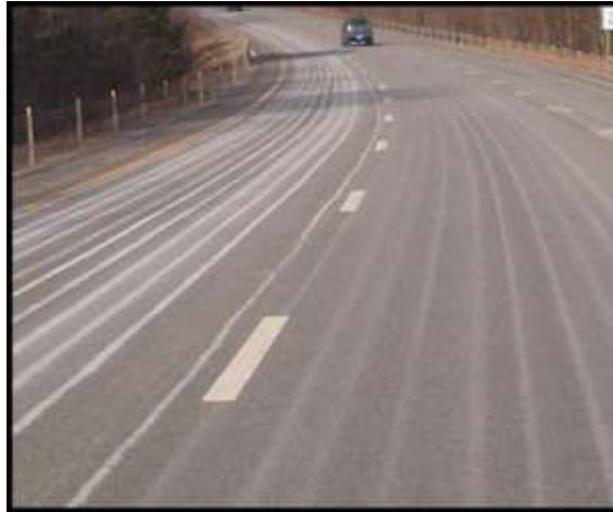
Figure 5: Pavement Pre-Treated with Sodium Chloride Brine Solution
