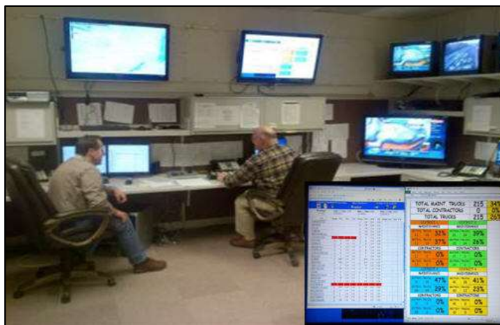
Figure 8: Activated Storm Center, Newington, CT.; (Insert) Storm Activation, Graphical Display
